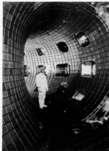
A worker stands inside the JT-60 machine during its recently completed renovation.
