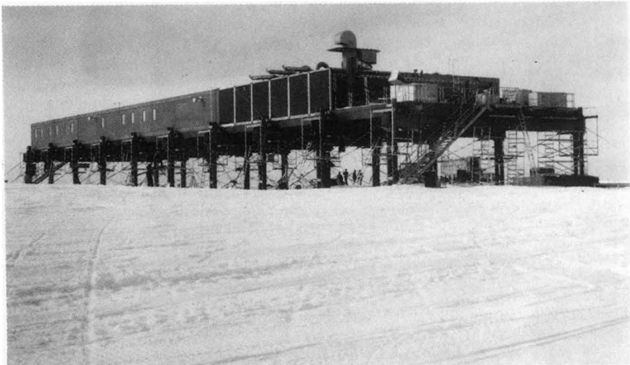
The new Halley base — science on stilts.
