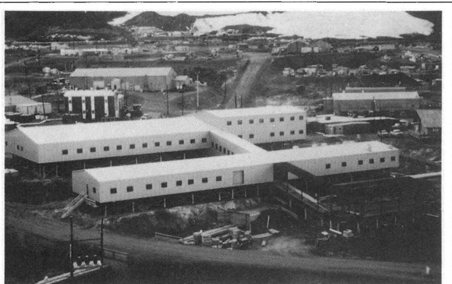
Nearly finished, in this October 1990 view, the new science laboratory at McMurdo Station. Cold Regions Research Laboratory photo by Wayne Tobiasson.
