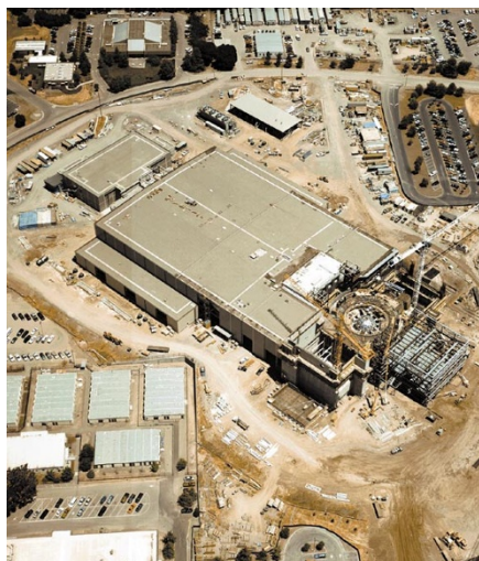
Costly: but NIF construction is proceeding steadily.
