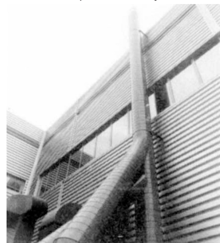
Raising the roof — an existing building extended to accommodate Celltech's new research centre.
