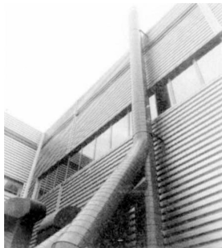
Raising the roof — an existing building extended to accommodate Celltech's new research centre.
