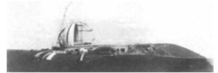
Dome completion soon.
