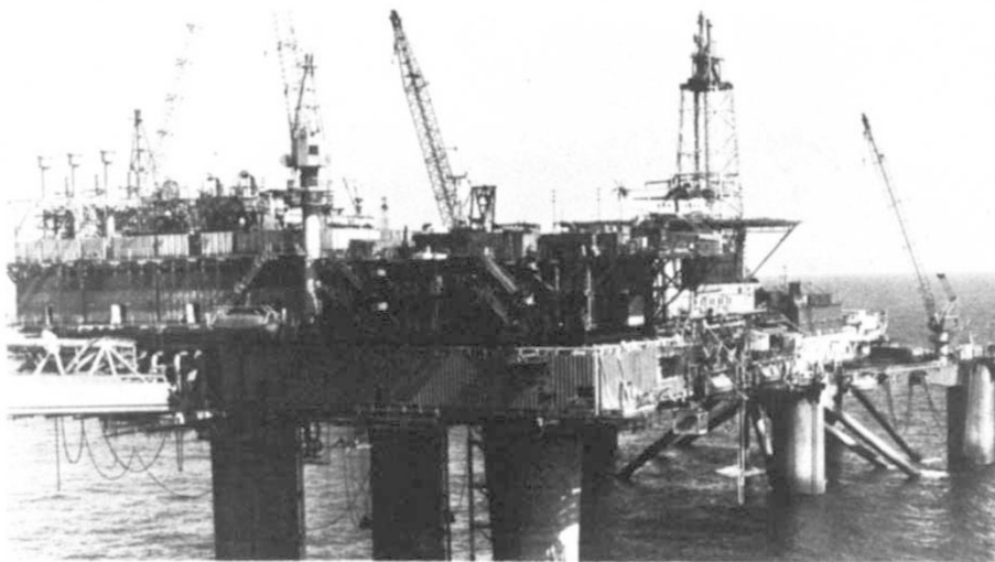
Energy from under the sea — a natural-gas rig in the North Sea
