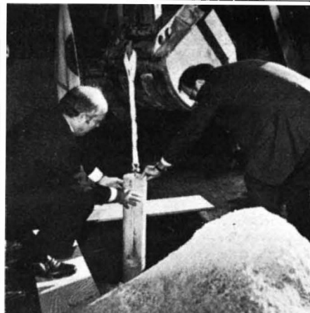
Laying the foundations for ISABELLE: has the US lost its initiative?
