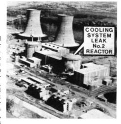
The accident resulted from an overheating of the core of the reactor causing some damage to the fuel rods. The emergency cooling system had flooded the core with water, but the contaminated water, some of which escaped through the roof of the plant as steam, was largely responsible for the escape of fission products such as xenon, krypton and iodine into the local environment.
