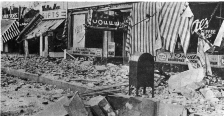
After an earthquake: devastation on the sidewalk of a southern California town.
