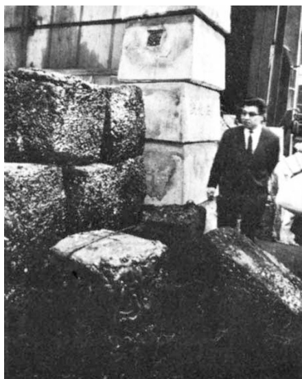
A constructive way of using waste: garbage crushed into blocks for use in the building industry.
