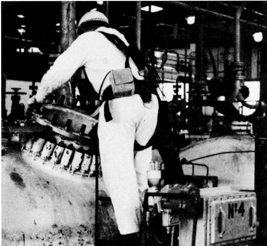
Preparing polymerisers for cleaning at BP factory.
