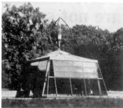
Solar collectors for heating
