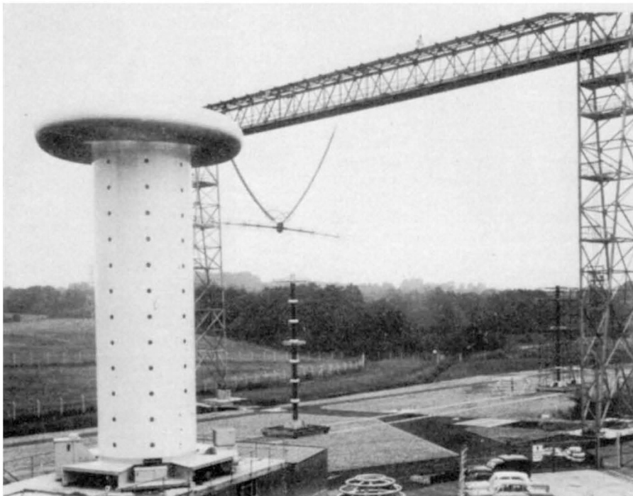
The CERL facilities at Leatherhead showing the Ferranti 5.2 million volt impulse generator and the test gantry that permits possible tower designs to be examined, and substation plant to be tested alongside. Eight conductors in a metre bundle are suspended from the gantry on the porcelain insulator strings.
