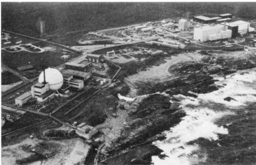
The Dounreay Experimental Reactor Establishment. The prototype fast reactor is in the right background, and the older Dounreay fast reactor is in the left foreground.
