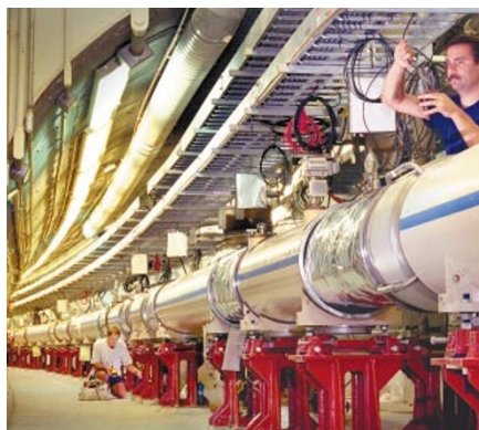
Collision course: rings have been placed inside a tunnel intended for ill-fated Isabelle accelerator.
