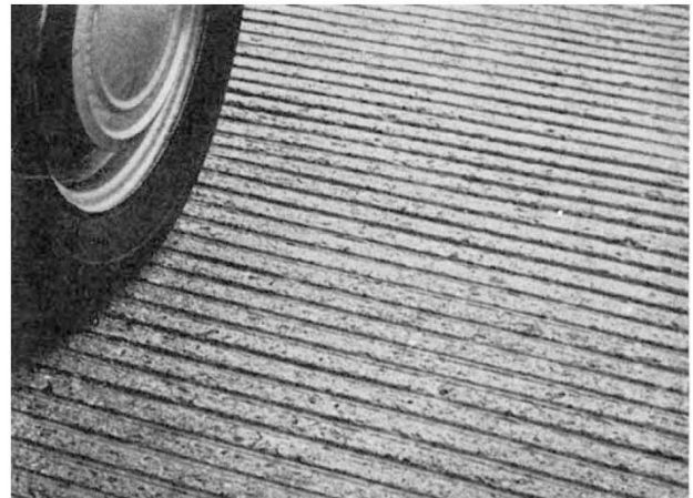
The addition of skid resistant texture to an existing concrete road.
