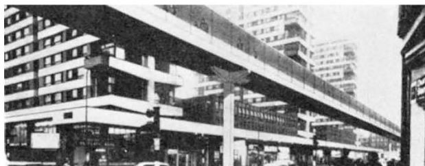
Photomontage of a Dunlop conveyor mounted above a city street. The whole structure weighs little, and support columns can be widely spaced.
