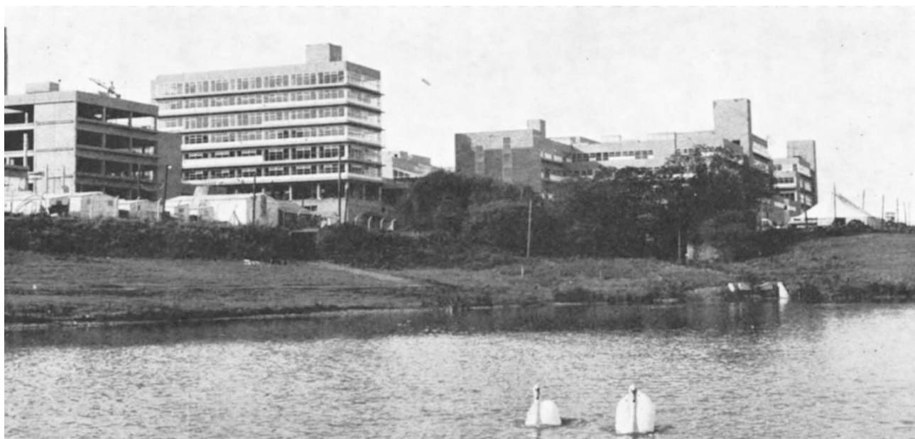
View of the university site from the north-east, showing Senate House, academic blocks of phase I (on right) and academic blocks of phase 2 under construction (on left).
