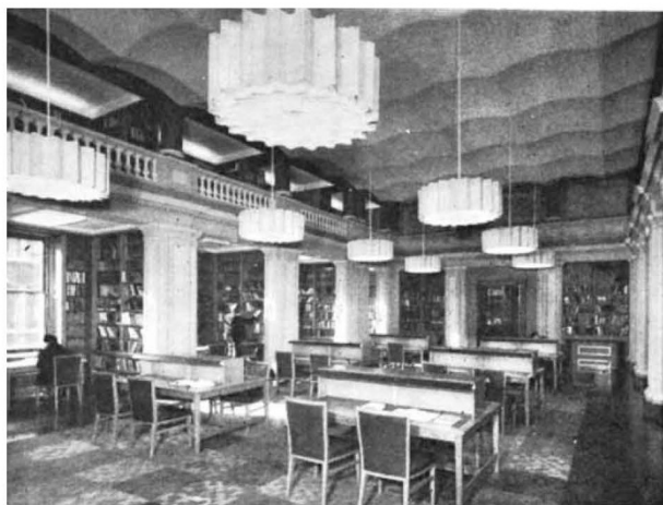
The library after conversion.
