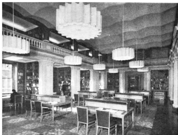
The library after conversion.
