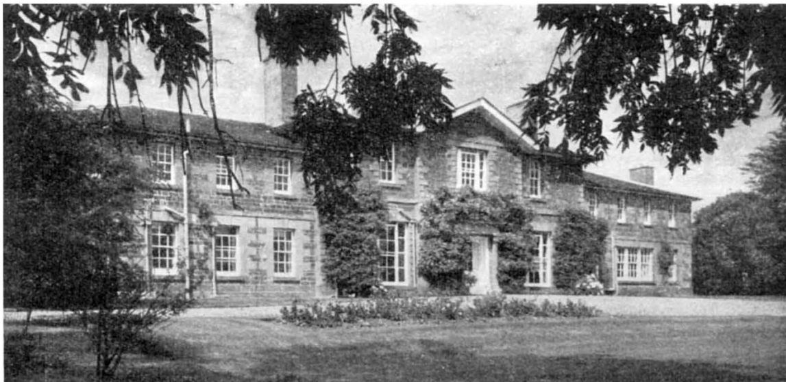
Fig. 2. Caswell House at the Allen Clark Research Centre of The Plessey Company, where research and development started in 1940
