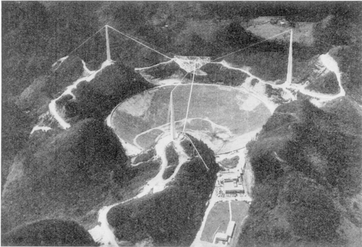
Fig. 2. Aerial picture of the giant radar radio telescope at Arecibo in Puerto Rico. The spherical dish antenna is 1,000 ft. in diameter and the movable feed arm is suspended on cables some 500 ft. above it from three concrete towers, two of which are 265 ft. in height and the third 365 ft.
