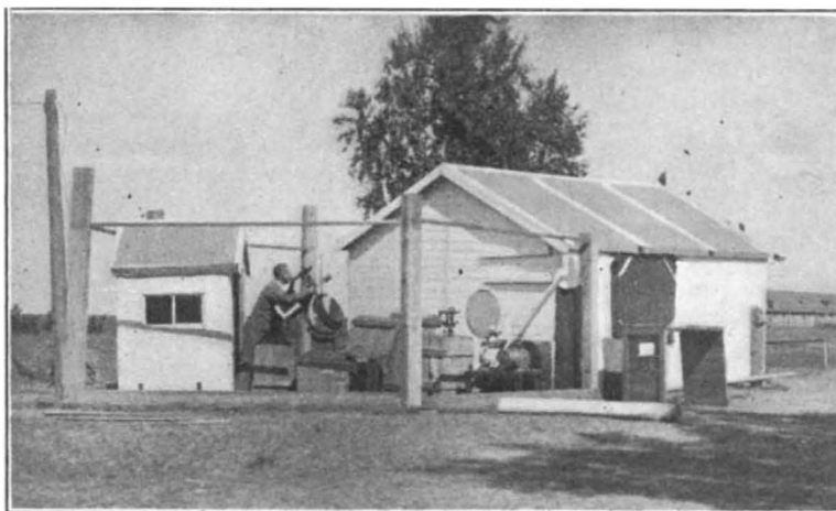
FIG. 1. Exterior of the cœlostât and experimental hut, looking east. The double-walled hut on wheels for sheltering the cœlostât is on the left. The larger hut is the double-walled, felt-lined hut for thermostatic sheltering of the instruments. At the nearest corner of the large hut can be seen the compressor for the refrigerator plant, and just above it the circular window to admit the horizontal beam from the cœlostât.
