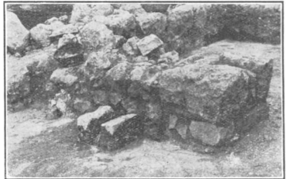
FIG. 4. West wall of residency lavatory and bathroom, showing sanitary fitting and, on left, drain from bath room.
