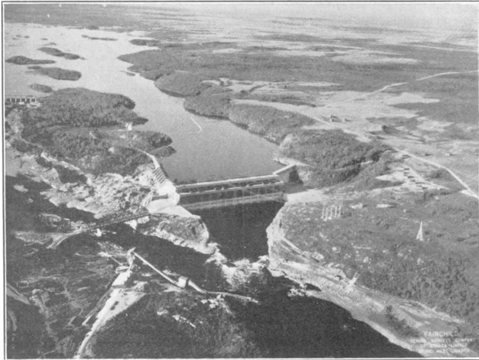
FIG. 1.—Hydro-electric installation (540,000 h.p.) at Isle Maligne, Lake St. John, Province of Quebec. (By courtesy of the High Commissioner of Canada.)
