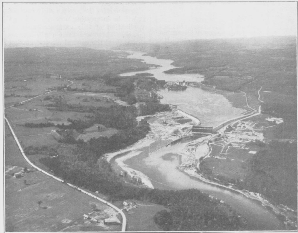
Fig. 2.—Two hydro-electric power stations on Gatineau River, Province of Quebec. Farmers' Rapids (120,000 h.p.) in foreground; Chelsea Dam (170,000 h.p.) beyond. (By courtesy of the High Commissioner of Canada.)
