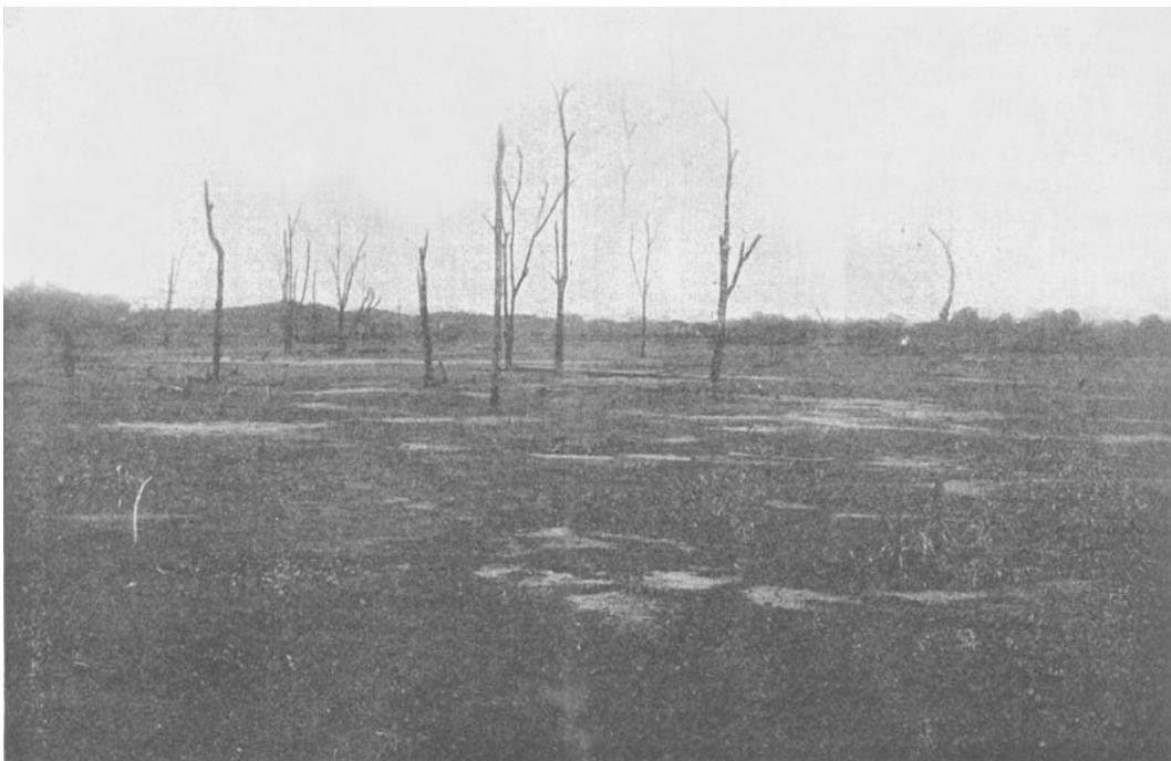
Land raised by "hydraulic filling" on the east bank of the French canal at Gatun. The remains of the swamp trees are still to be seen. From "Rural Sanitation in the Tropics."
