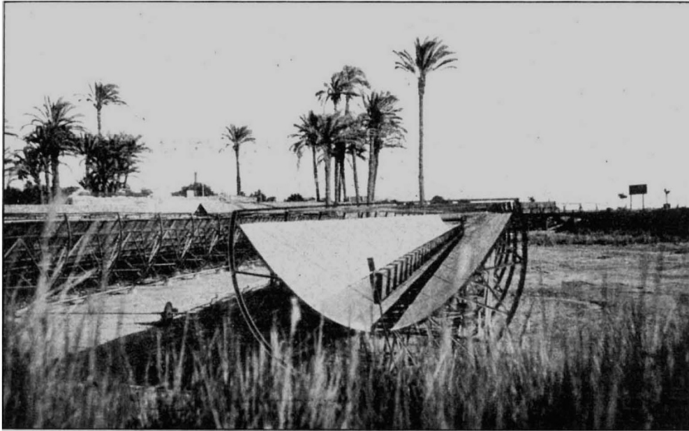
FIG. 2.—Shuman-Boys absorber, Meadi, 1913. One section of the absorber from the north.
