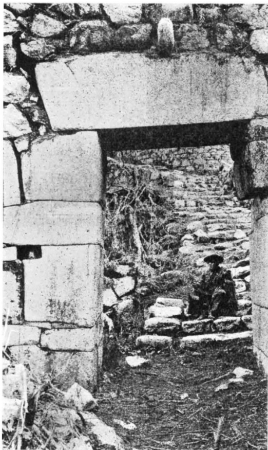
FIG. 5.—Machu Picchu. City gate, interior. Notice the lock hole containing granite cylinder on left and projecting ring stone over the lintel of the doorway. The gate, probably of wood, was either swung from the ring stone or fastened to it and balanced by a log fastened to the stone cylinders in the lock hole on either side of the gateway. A similar device was used also in the entrance doors to each isolated group of houses. Copyright by the National Geographic Society.
