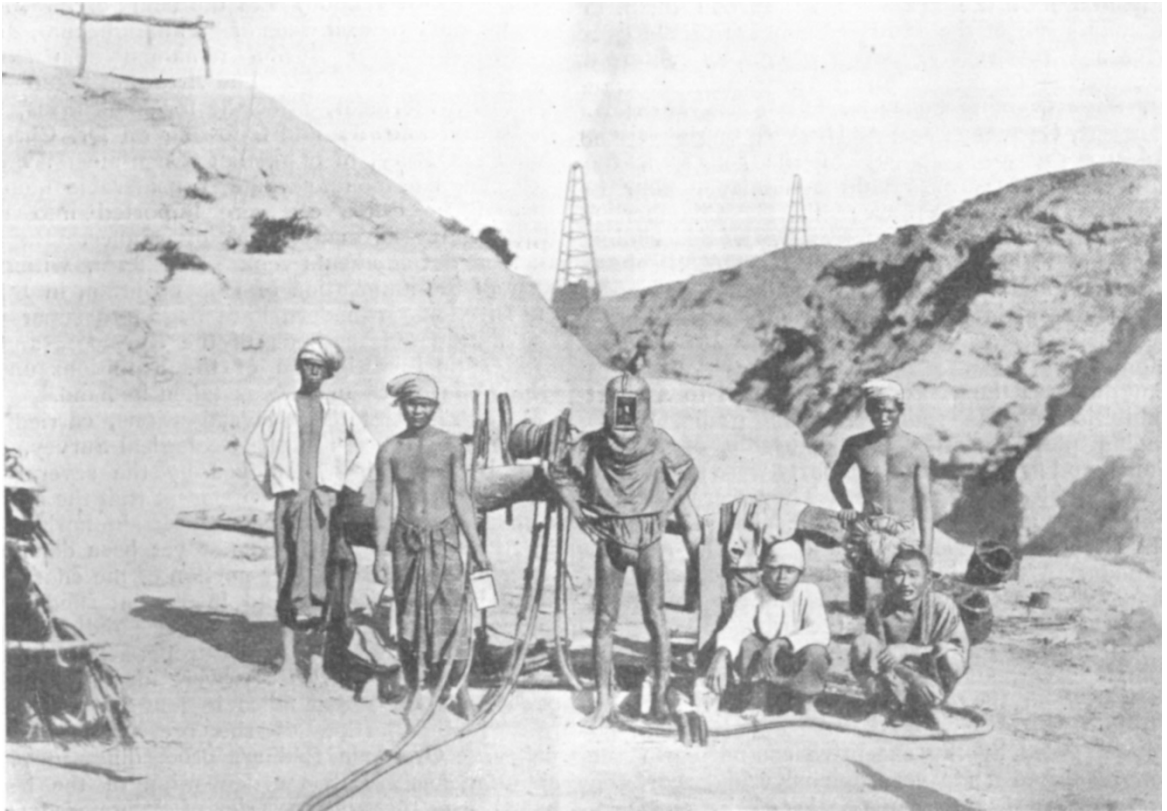
Yenangyaung—Native well-digger in diving dress. (The man on his right is holding the mirror used to illuminate the bottom of the well.) From Memoirs of the Geological Survey of India , vol. xl., part i., "The Oil-fields of Burma."
