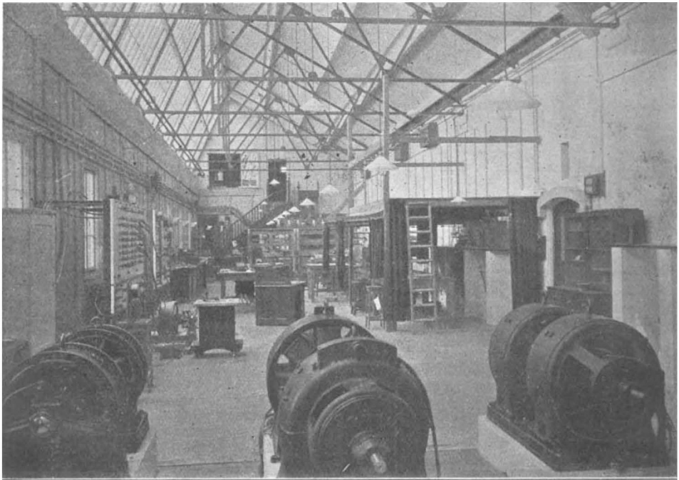
FIG. 1.—General view of large bay of Electrotechnical Building, looking east.
