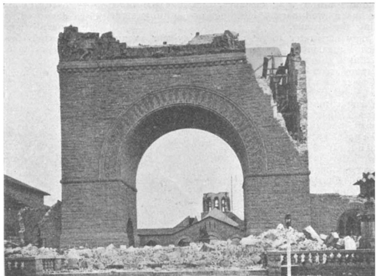
FIG. 2.—Memorial Arch, Leland Stanford Junior University. Earthquake Effect:—The beams designed to stiffen the walls were not tied to them, and helped to batter them down when the shock came. (Photograph by Richard L. Humphrey.)
