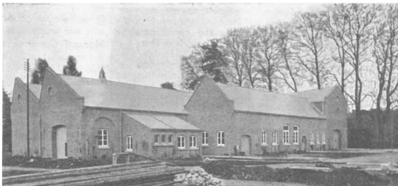
FIG. 1.—New Buildings of the National Physical Laboratory.
