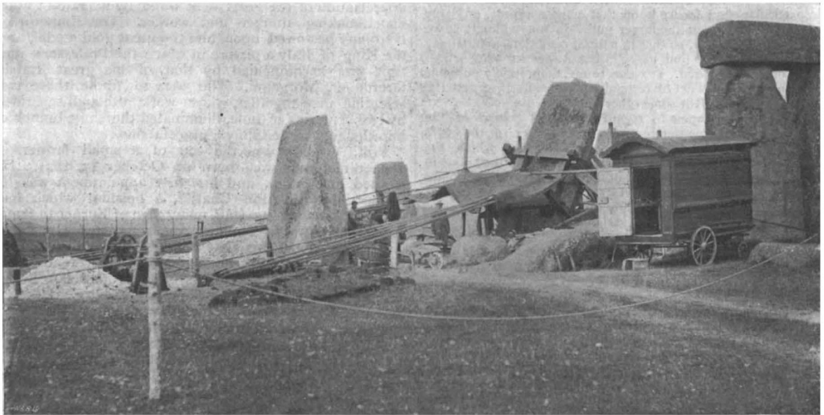
FIG. 1.—The work at Stonehenge. Raising the leaning stone.
