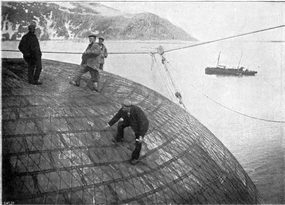
FIG. 1.—The top of the balloon, showing the joinings of the pieces.
