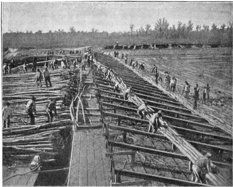
FIG. 2.—Constructing Fascine Mat on Mattress Ways
