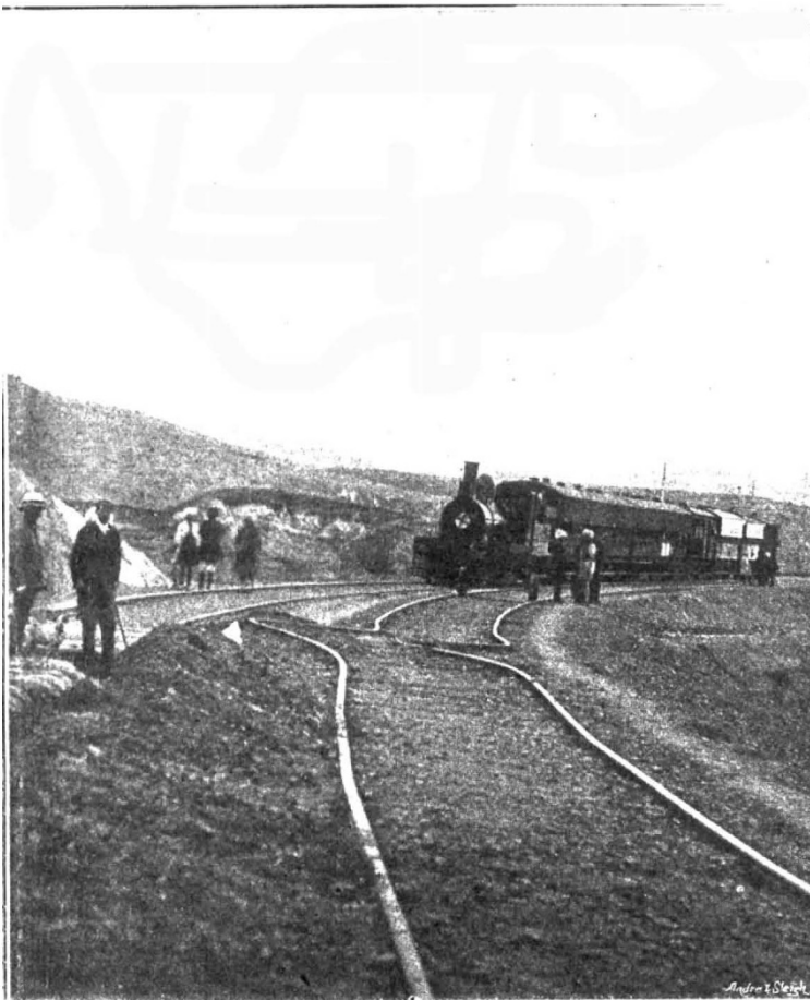
View showing distortion of rails caused by earthquake between Sanzal and Old Chaman.
