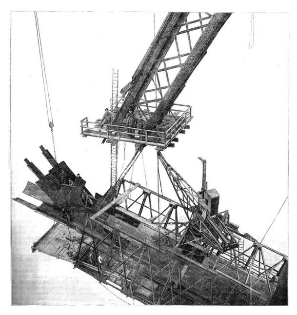
less than the connection of the web of a lattice girder with one of its booms, but here the junction alone weighs as much as an ordinary iron railway bridge of 100 feet span. This mass of steel work is suspended 80 feet above high water, and projects 180 feet beyond the masonry piers. Considerable forces are sometimes needed to bring the tubes into their correct position; and as in the case of the Britannia Bridge, which on a hot day moves 3 inches
