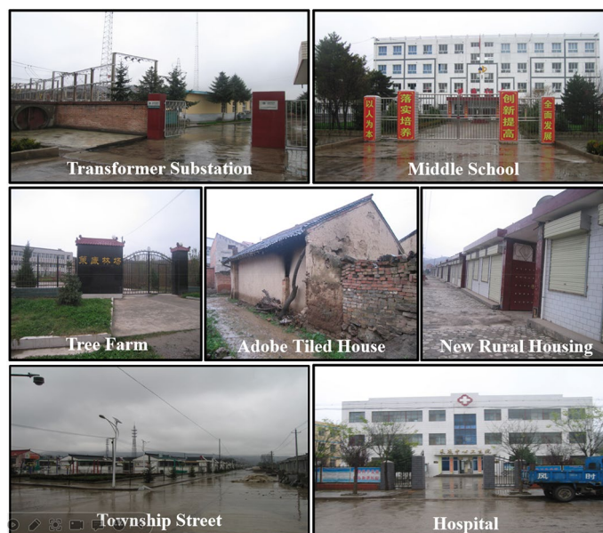
Figure 1. Representative buildings on the surface section.
