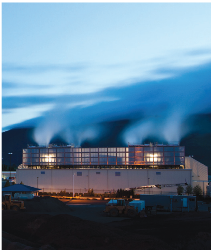
Steam carries heat away from Google's data centre in The Dalles, Oregon.
