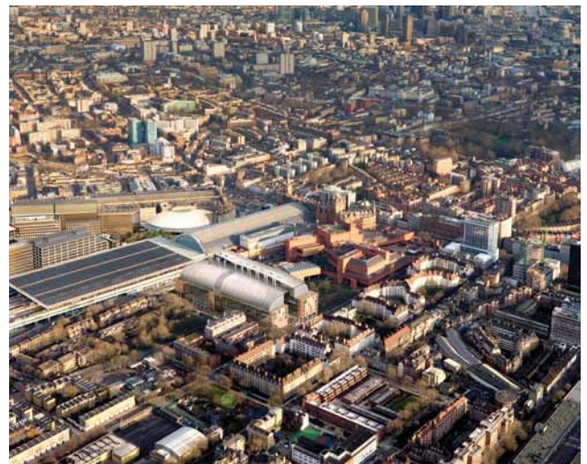
Aerial view of the proposed building and the surrounding area. © Cityscape
