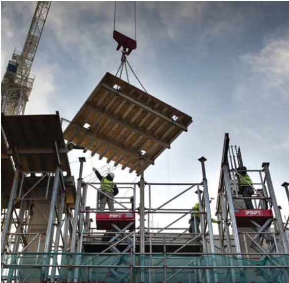
The Crick under construction. © Wellcome Images
