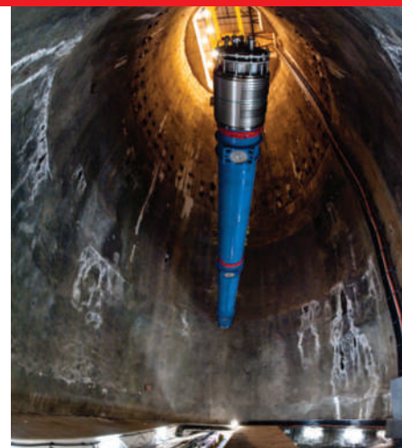
A superconducting magnet is removed at the LHC.
