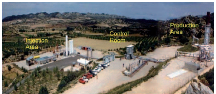
A UGC trial facility at El Tremedal in northeast Spain in 1998.
