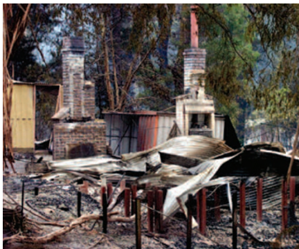
Fig. 1 A home in ruins (photograph with permission – Rob Carew)
