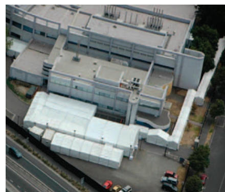
Fig. 5 Victorian Institute of Forensic Medicine and Coronial Services temporary mortuary facility, showing marquee and security fencing in place and refrigerated containers (photograph with permission – VIFM)
