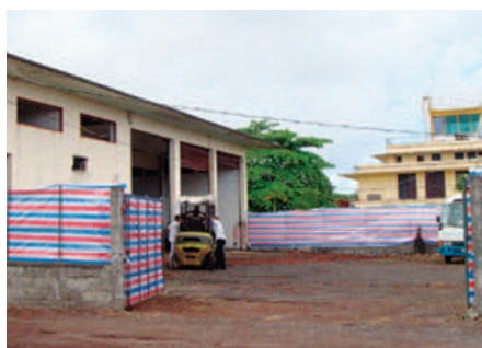
Fig. 3 Disused fire station at an old airport used as temporary mortuary in Moroni, Comoros Islands (with permission of Blake Emergency Services)
