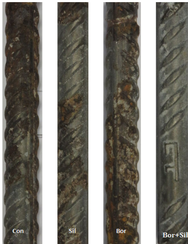
Figure 14. Images of rebar samples embedded in different mortars (Con = control; Sil = silicate; Bor = borate; Bor + Sil = borate + silicate) and removed after 43 cycles of wet/dry treatments.
