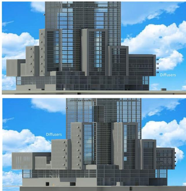
**Figure 9.** Several optimized diffusers with an area ratio of 1.5 fixed to sides of facades of a tall building development.
