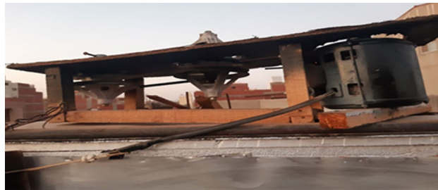
Figure 5. Trolley rotation control unit.
