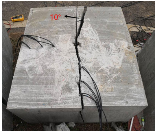
Figure 13. Blast-induced crack distribution in Model 2.
